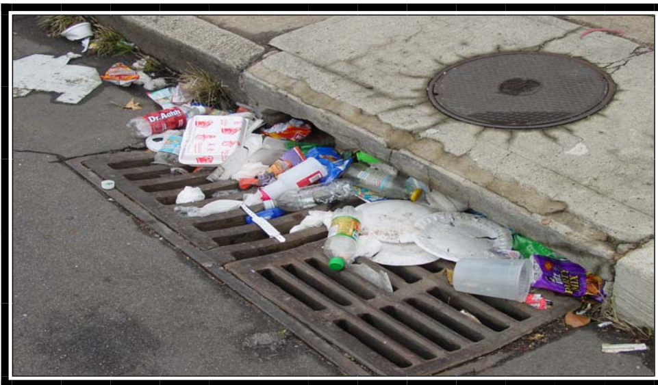
Litter, including plastic beverage bottles, is washed down storm drains, flows into streams, into the Baltimore Harbor, and out into the Chesapeake Bay.
